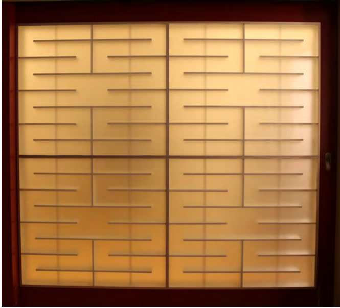
Figure 1: Metamaterial wall in the recording studio as four labyrinth structures (four-panel). In the studio two such walls are present next to each other movable sideways.
